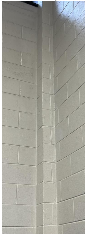
Gymnasium Corner AFTER repair
